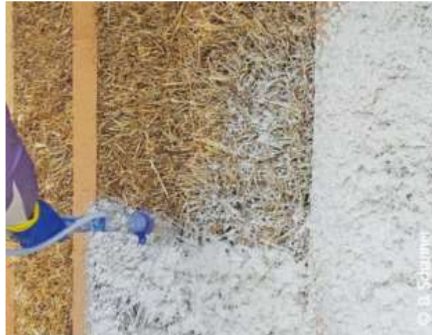
Lime plasters on straw balls
