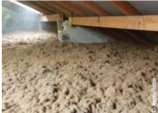
Seaweed insulation on top floor
