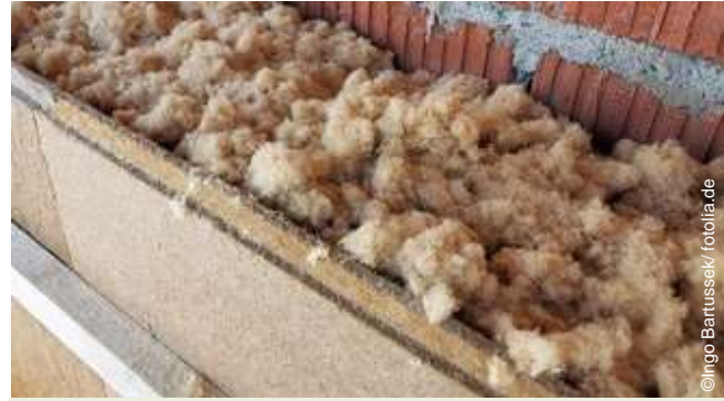
Cellulose insulation wool
